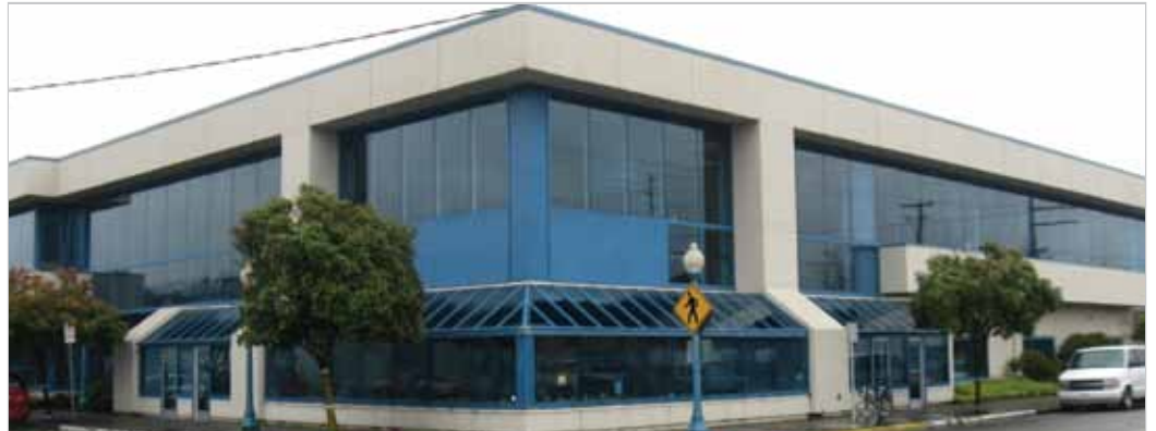
In 2011 Ameresco completed a comprehensive $2.7 million Energy Savings Performance Contract (ESPC) for the City of Olympia, which updated aging infrastructure to reduce energy and water consumption.
